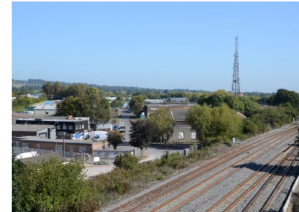
URBAN, the railway running alongside the Crown Industrial Estate.
